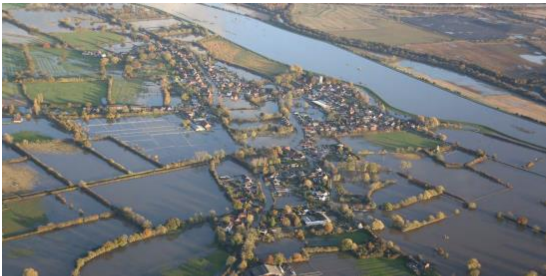
Figure 6. Flooding at Fishlake during the 2019 flood event
