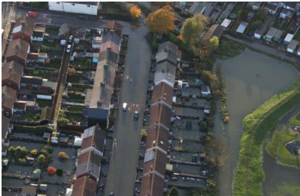
Figure 7. Flooding at Bentley during the 2019 flood event.
