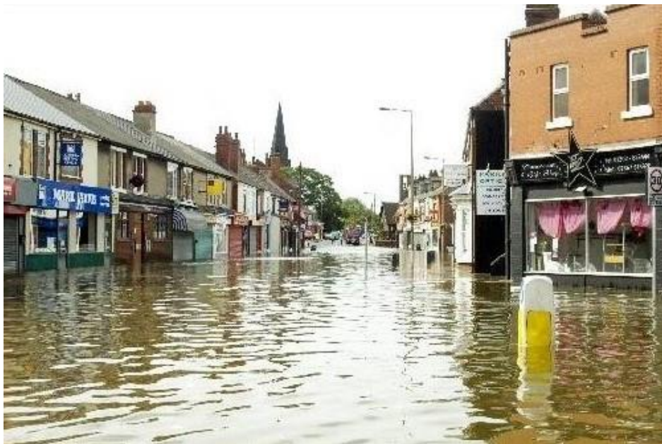
Figure 5. Bentley High Street during the 2007 flood event.
